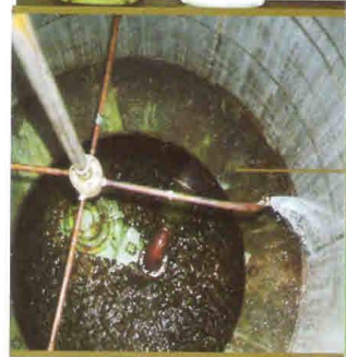
SEWER OVERFLOWS CDS gross solids separator used to screen sewer overflow at relief point. All visible solids removed before discharge.
