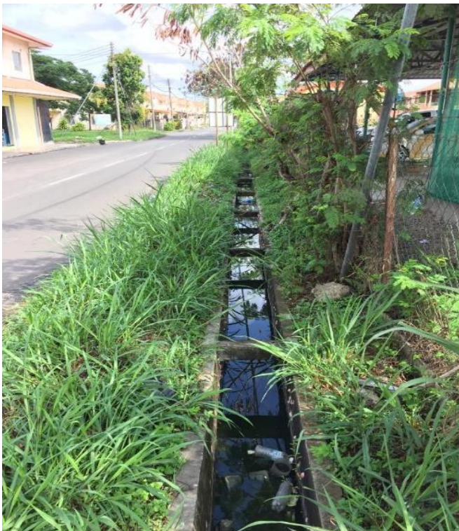
Photo 3.3 Picture of drain outlet from Taman Miramas
