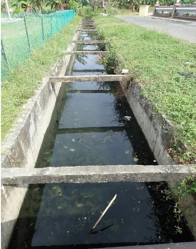
Photo 5.1 Example of drain topographic survey conducted at Taman Miramas
