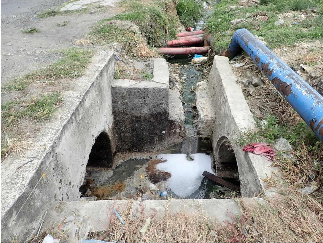
Photo 5.3 Example of culvert structure survey conducted along Jalan Hospital (Catchment S2)
