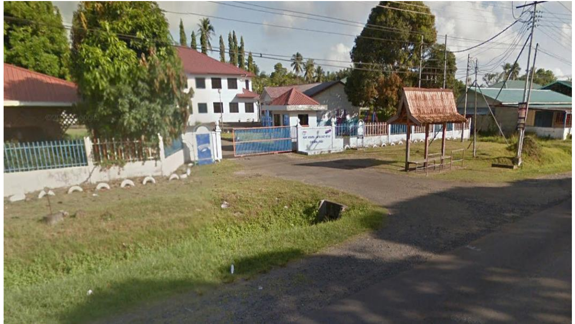
Photo 3.12 Picture of earth drain in front of Pejabat KEMAS along Jalan Balung-Semporna
