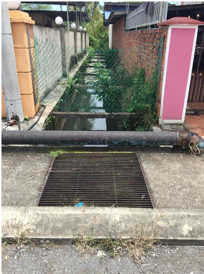
Photo 3.1 Example of a concrete lined channel located within the study area (Housing drain within Taman Miramas, facing downstream)
