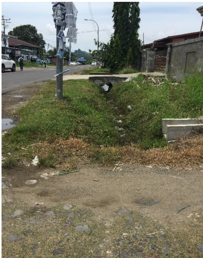
Photo 3.5 Picture of drain along Jalan Kabongan
