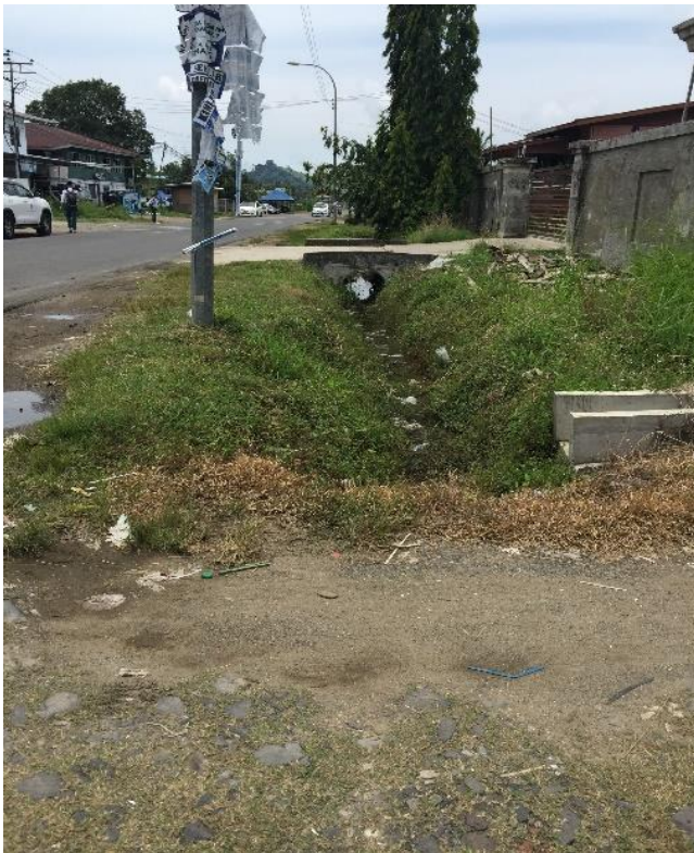
Photo 5.2 Example of drain topographic survey conducted along Jalan Kabongan
