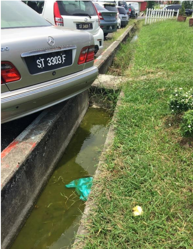
Photo 3.6 Picture of a concrete drain in front of Kolej Poly-Tech Mara
